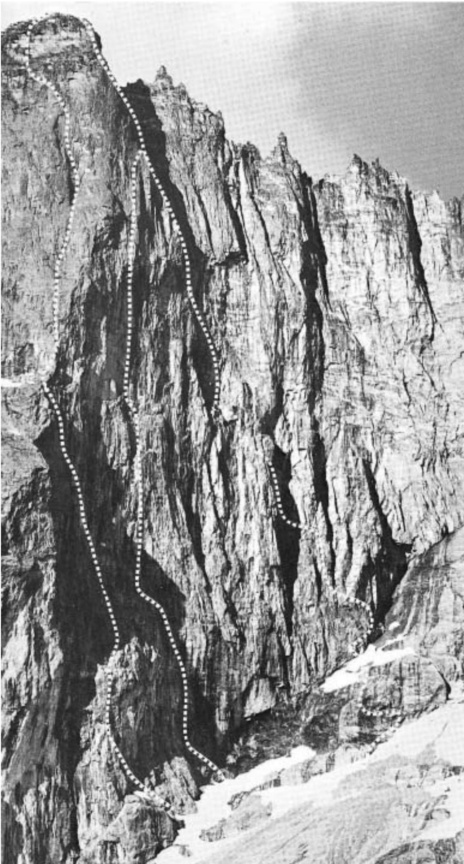
The 5000 foot Trolltind Wall ("Trollveggen") with: 1. Norwegian Route, 1965, 2. English Route 1965, 3. French Route 1967. H. Sodahl
