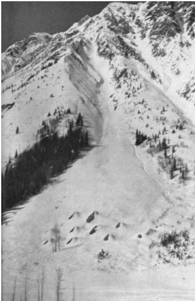
Figure 5. Earth Mounds At The Bottom Of An Avalanche Path. Photo Bruno Engler (More mounds are to be built on the right side.)
