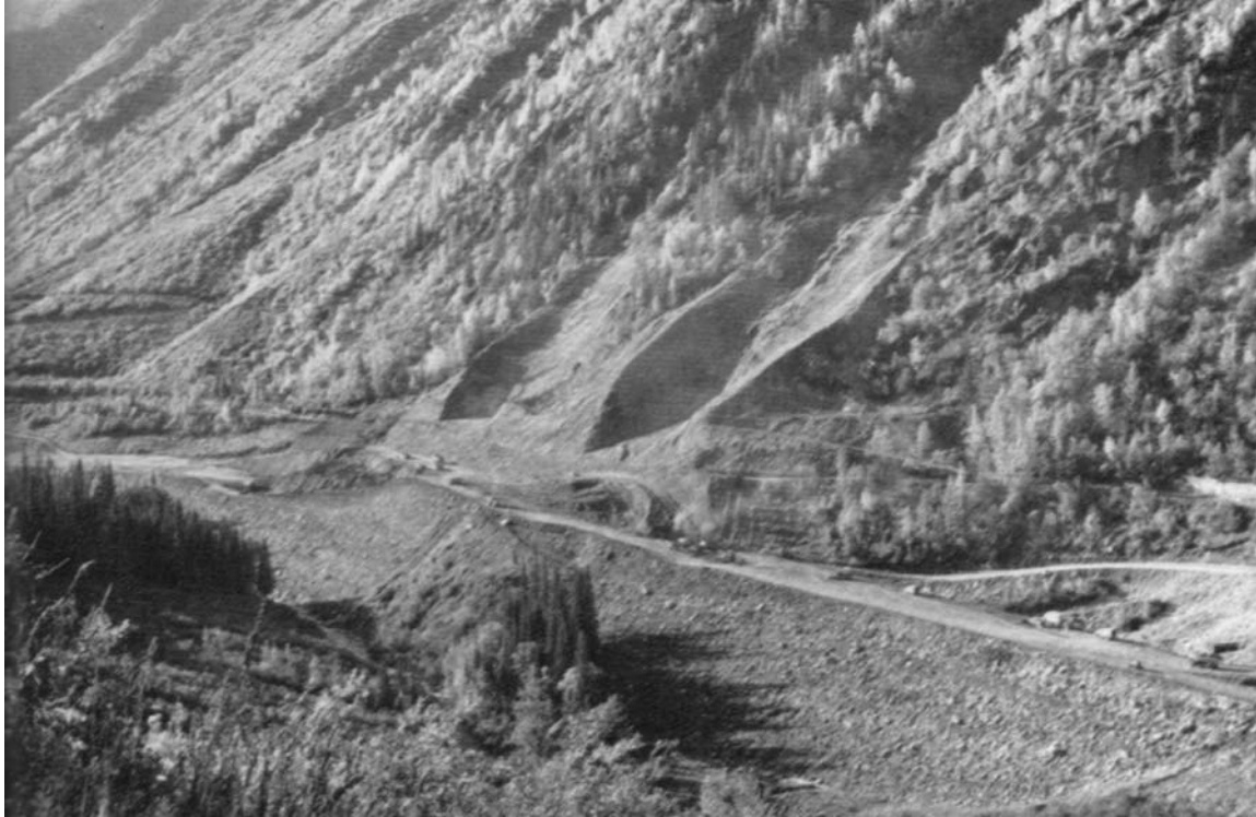
Figure 4. Dams And Excavated Channels For The Avalanches At Mt. Tupper. Photo Division Of Building Research, NRC.
