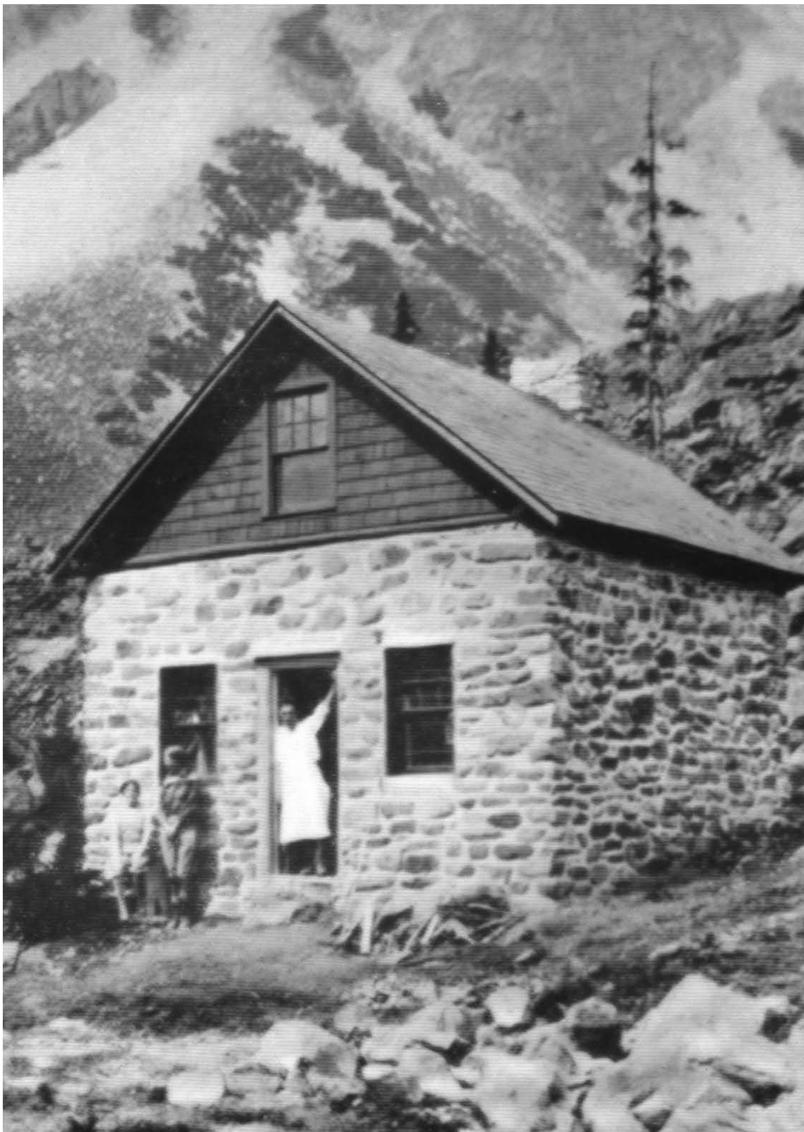
The Memorial Cabin. Photo C.G. Wates
